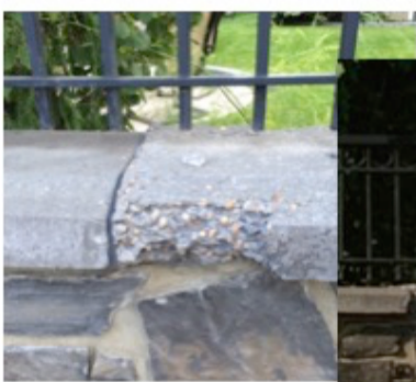
Stone Feature Repair
